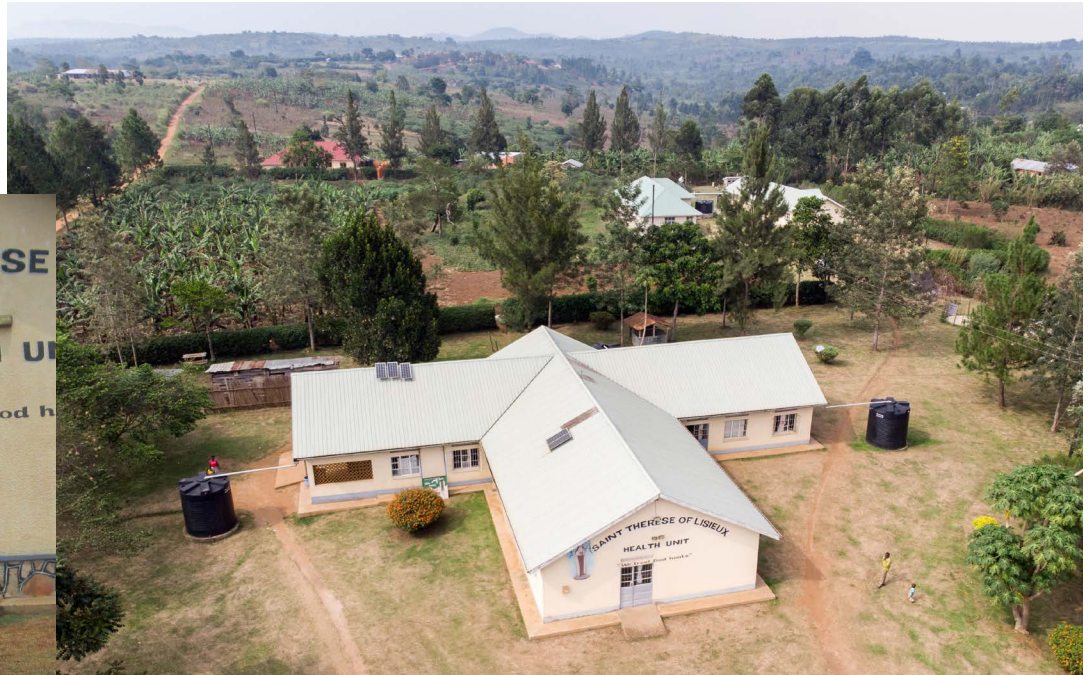
Rwibaale Hospital, Uganda
